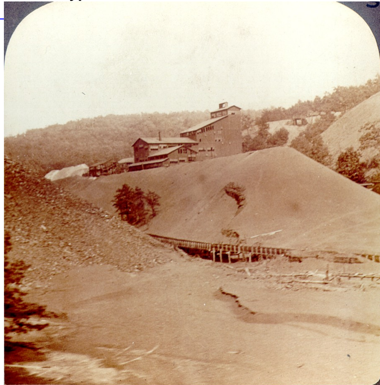
11241 - Typical coal breaker with culm heaps, anthracite fields Pennsylvania. Copyright Underwood & Underwood, U-54612
